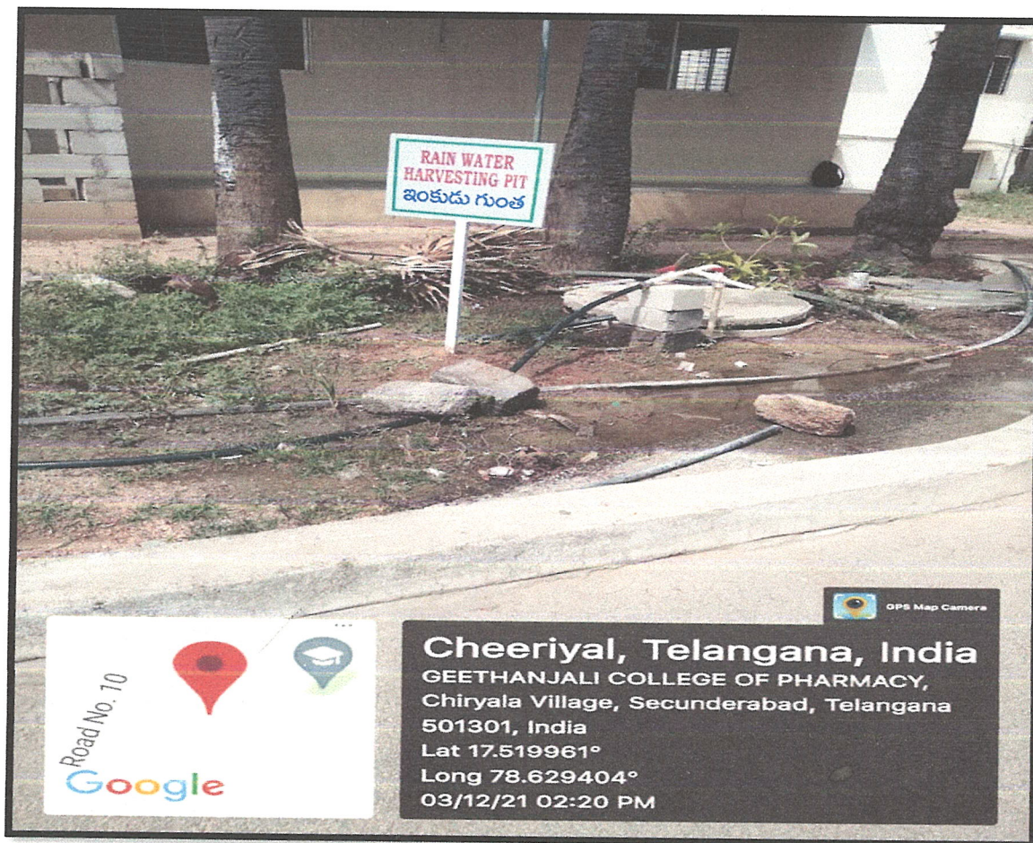
Rain water harvesting pit
